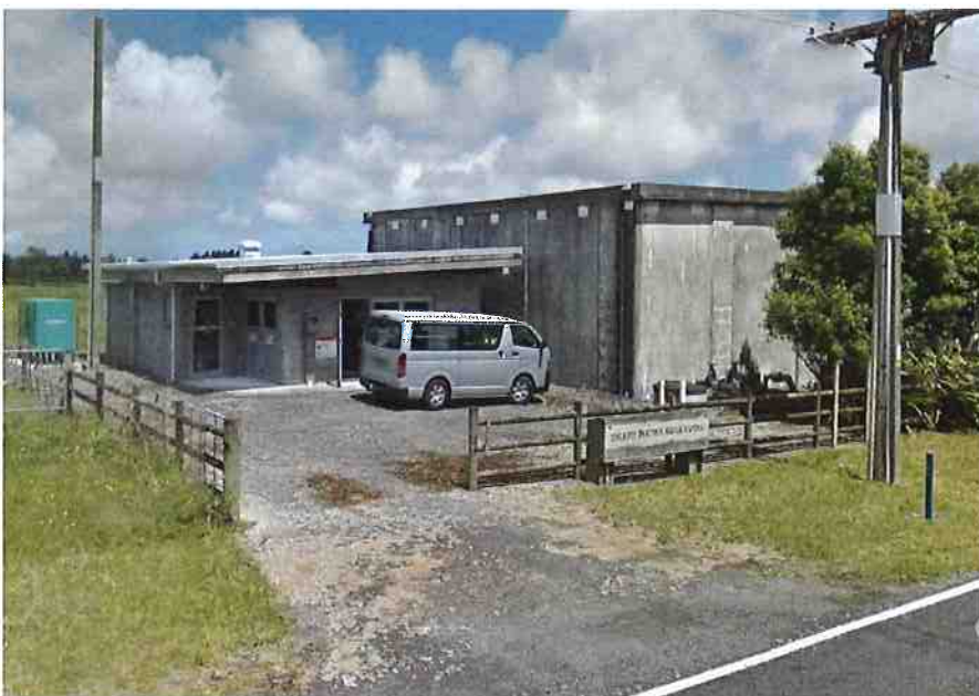
Figure 3: Okato water treatment plant as viewed from Oxford Road facing west (Google Maps)
