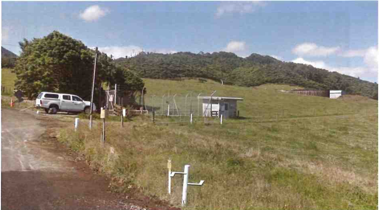
Figure 2: View of reservoir water booster pump building in center and reservoir and Oakura Water Treatment Plant building on right in distance as viewed from Wairau Road. Wire fencing in center is not associated with this asset (Google Maps)
