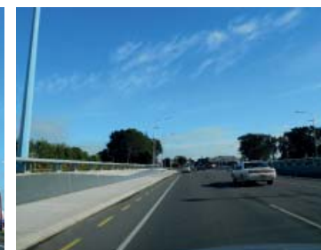
G. The Vickers to City project has been completed with a new city bound bridge over the Waiwhakaiho.
