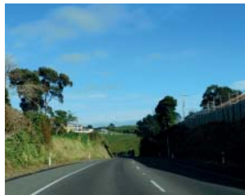
C. The road cutting at the 50km threshold is not currently included in the entrance corridor.
