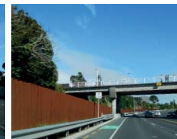
H. In the past 4 years vegetation removal has been undertaken in places. It is replaced with a corten steel fence on the Parson Street underpass.
