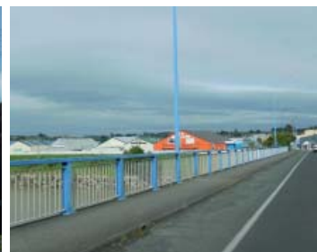
H. The Waitara River Bridge is an important threshold marking the arrival to the town centre.
