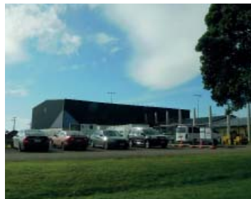
C. The Waitara Gymnasium has been recently constructed on Clifton Park.
