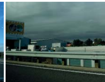
D. The industrial storage sheds and billboard illustrate the outcome when there is no planting or screening.
