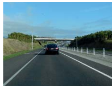
B. The planting is established at the Henwood Road overpass.
